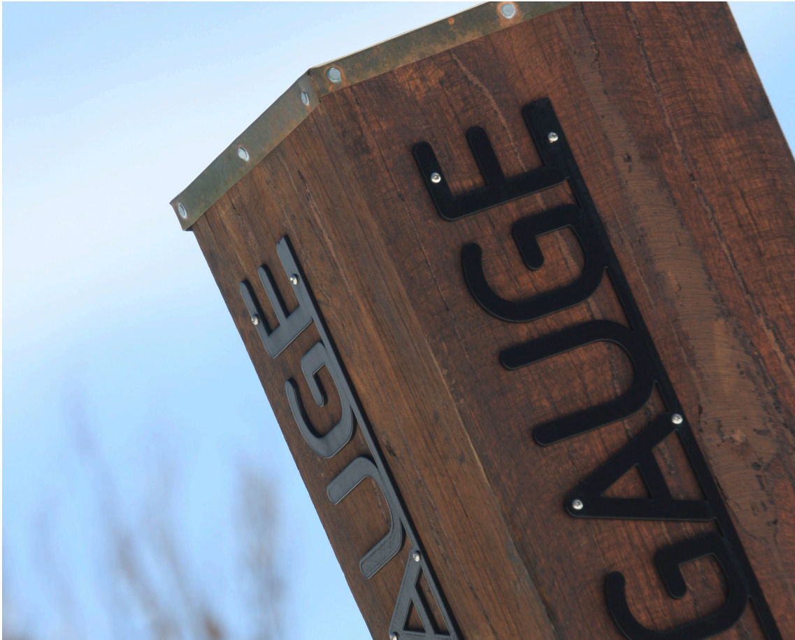
Top: Detail of weather resistant copper plate cap, Bottom: Detail of vitreous enamel sign plate
