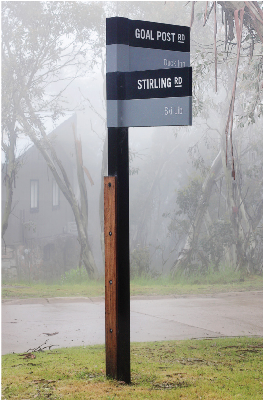
Left: Typical wayfinding sign with detail of red gum timber dressing, Right, Detail of wayfinding graphics.
